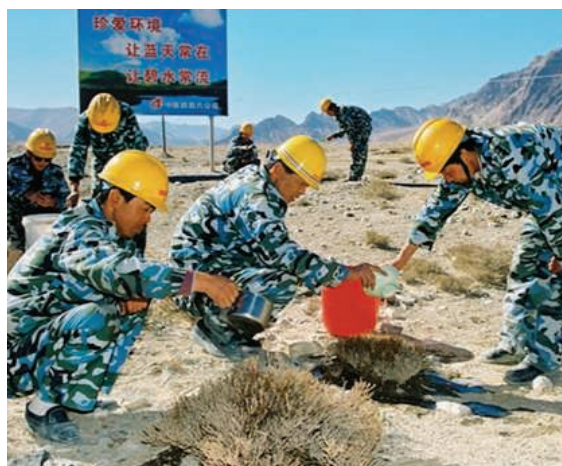
Grass restored. Grassland vegetation and its root soil layer were removed during construction then were replanted once the work was complete (12).
